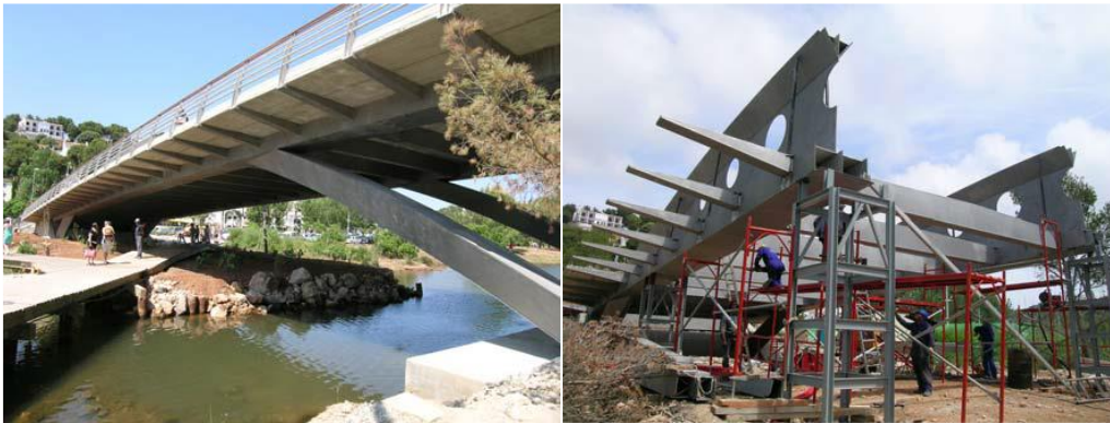
Fig. 2. Cala Galdana Bridge, Final phase (left), construction phase (right). [8]
