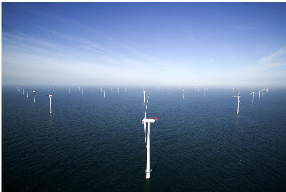
Figure 1.2: Photograph of Horns Rev I wind farm, where we can see the type of off-shore windmill we will be considering in the present project: 3 blade off-shore windmill with a hub height of approximately 65 meters above sea level and a 2 MW power ( source: http://nortus.pinger.pl/m/2173121 ).
